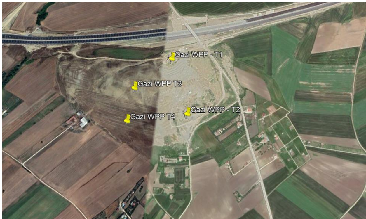
Figure 2. Location of Turbines of Gazi Wind Power Plant
