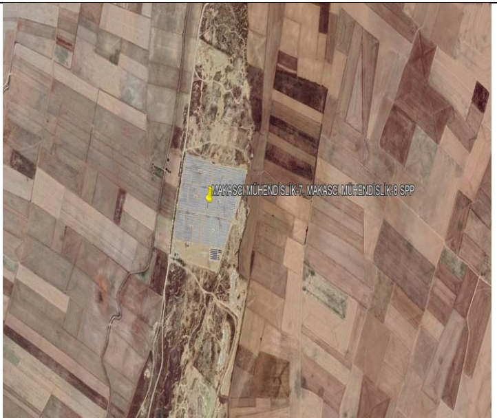
Solar Installation Verification. & Location Verification
