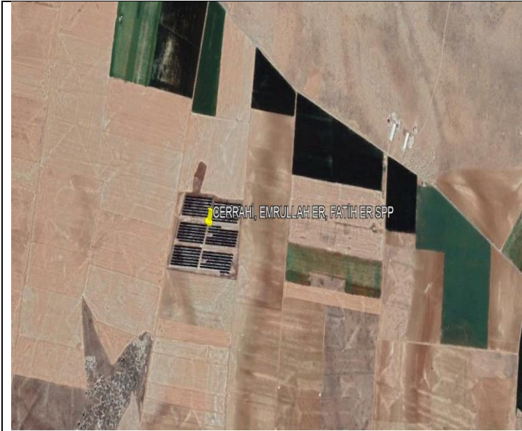
Over all view of Project Installation
