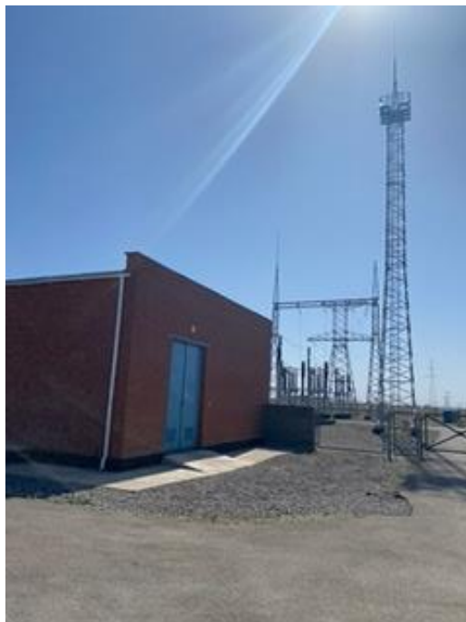
The substation of the project
