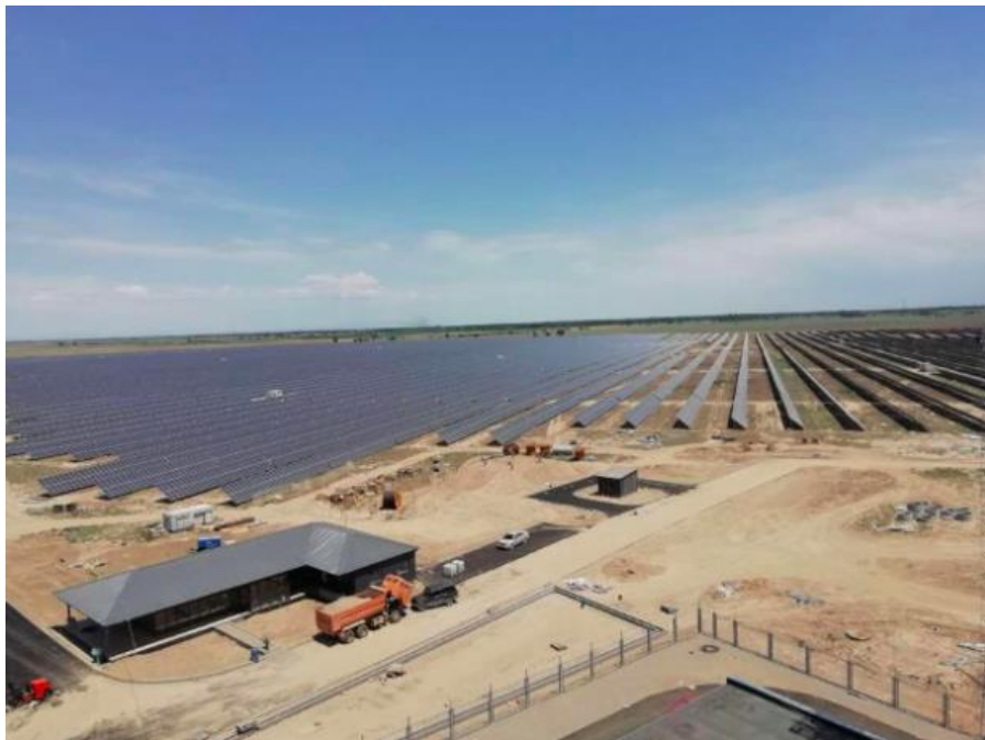
The overview of all PV arrays
